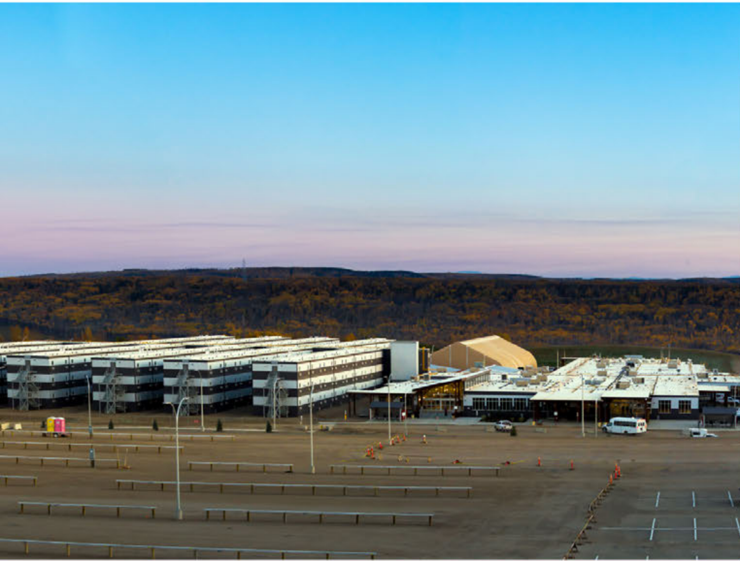
Two Rivers Lodge, B.C. Hydro Site C
