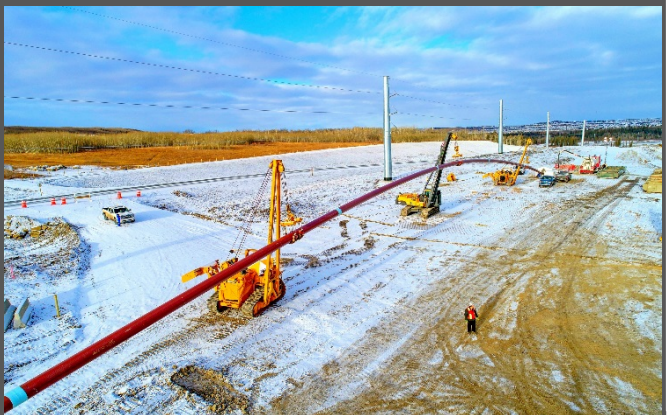
NATURAL GAS TRANSMISSION $297M
