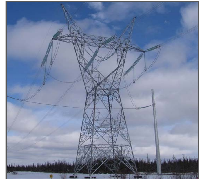
FORT MCMURRAY WEST 500 KV TRANSMISSION
