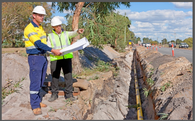
INTERNATIONAL NATURAL GAS DISTRIBUTION $92M
