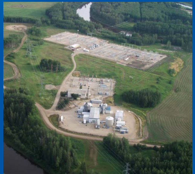
The Valleyview Generating Station was part of the fossil fuel-based generation portfolio sold in September 2019.
