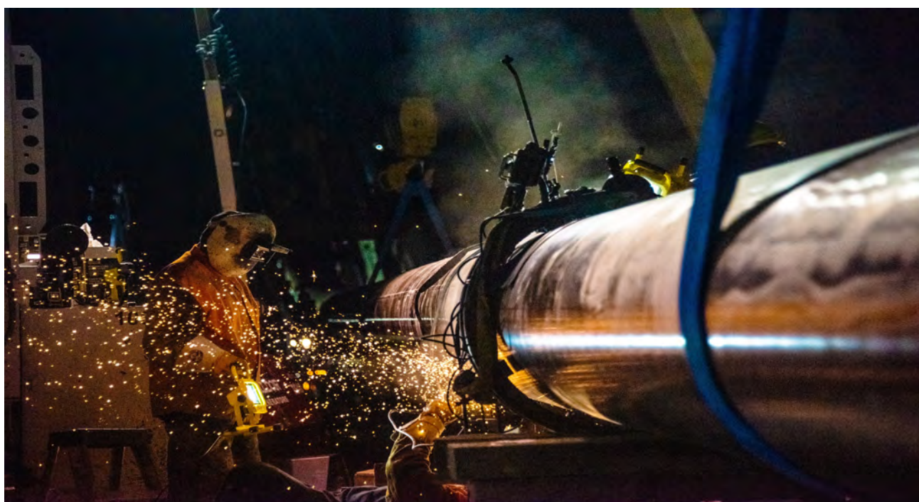
Pembina-Keephills transmission pipeline construction, near Wabamun Lake, Alberta
