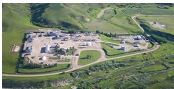
Natural gas storage facility, Carbon, Alberta
