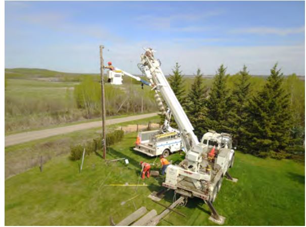
Electricity Distribution, Maintenance Work, Alberta
