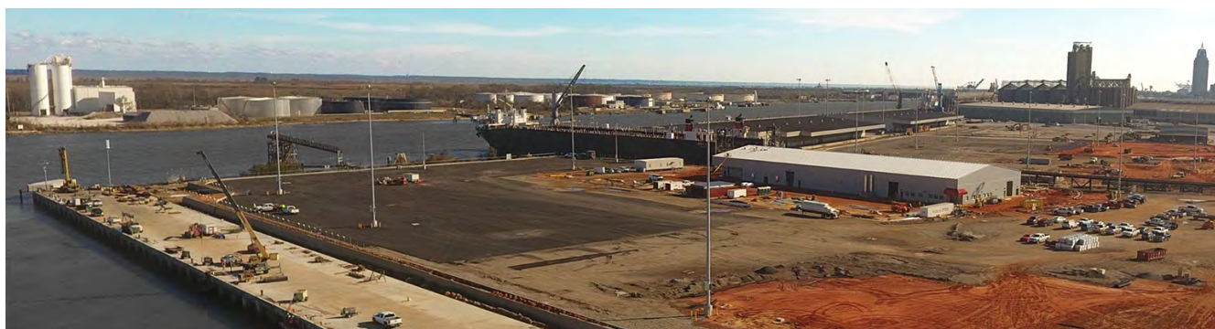
Construction Site of RoRo terminal, Mobile, Alabama
