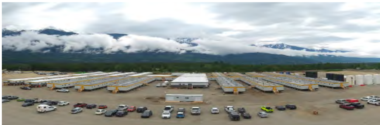
Trans Mountain Expansion Project Camp, Valemount, British Columbia
