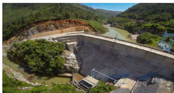
Hydroelectric power station, Veracruz, Mexico
