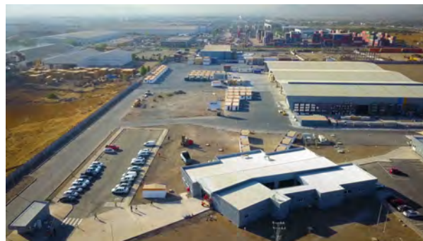
ATCO Sabinco, Manufacturing Facility, Santiago, Chile
