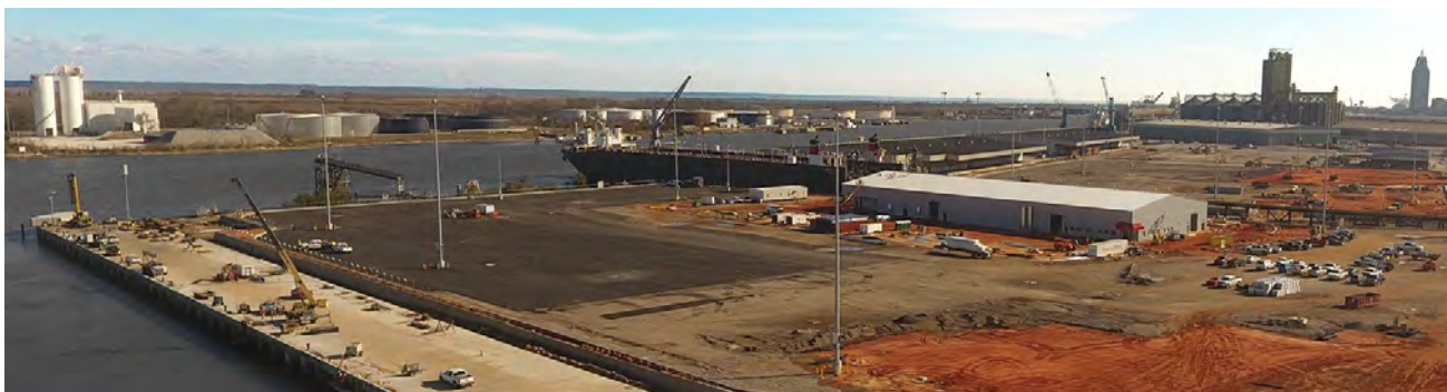
Construction Site of RoRo terminal, Mobile, Alabama
