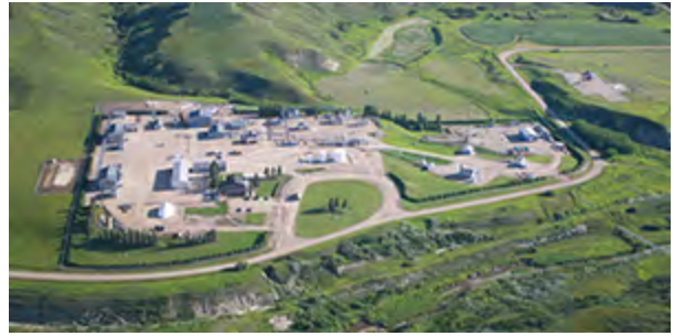
Natural gas storage facility, Carbon, Alberta
