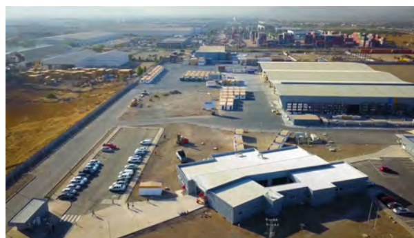
ATCO Sabinco, Manufacturing Facility, Santiago, Chile
