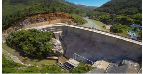
Hydroelectric power station, Veracruz, Mexico
