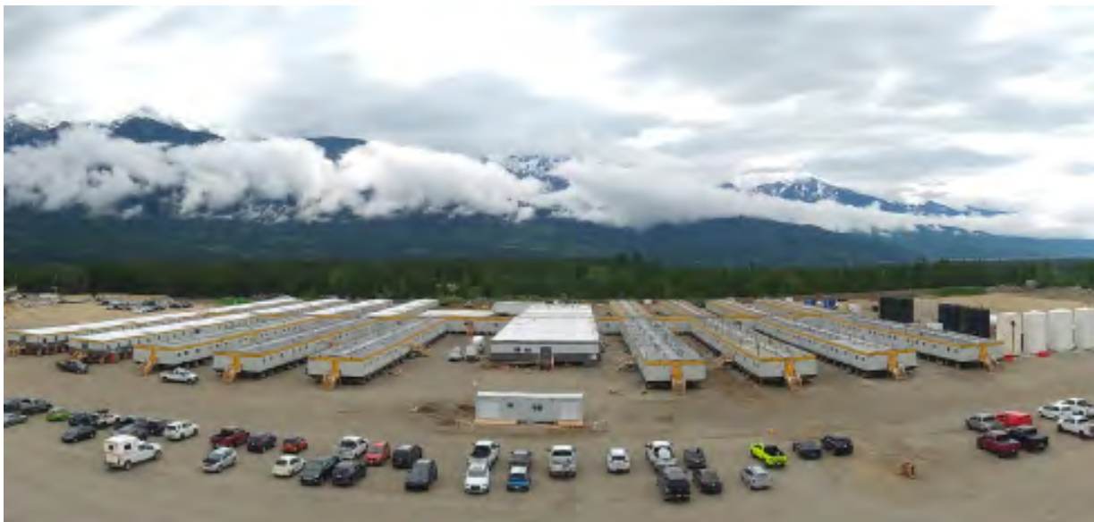
Trans Mountain Expansion Project Camp, Valemount, British Columbia
