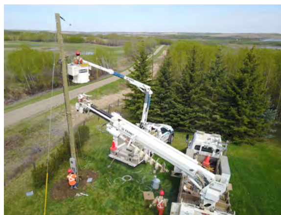
Electricity Distribution, Maintenance Work, Alberta
