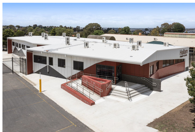
Hallam Primary School, Victoria Australia
