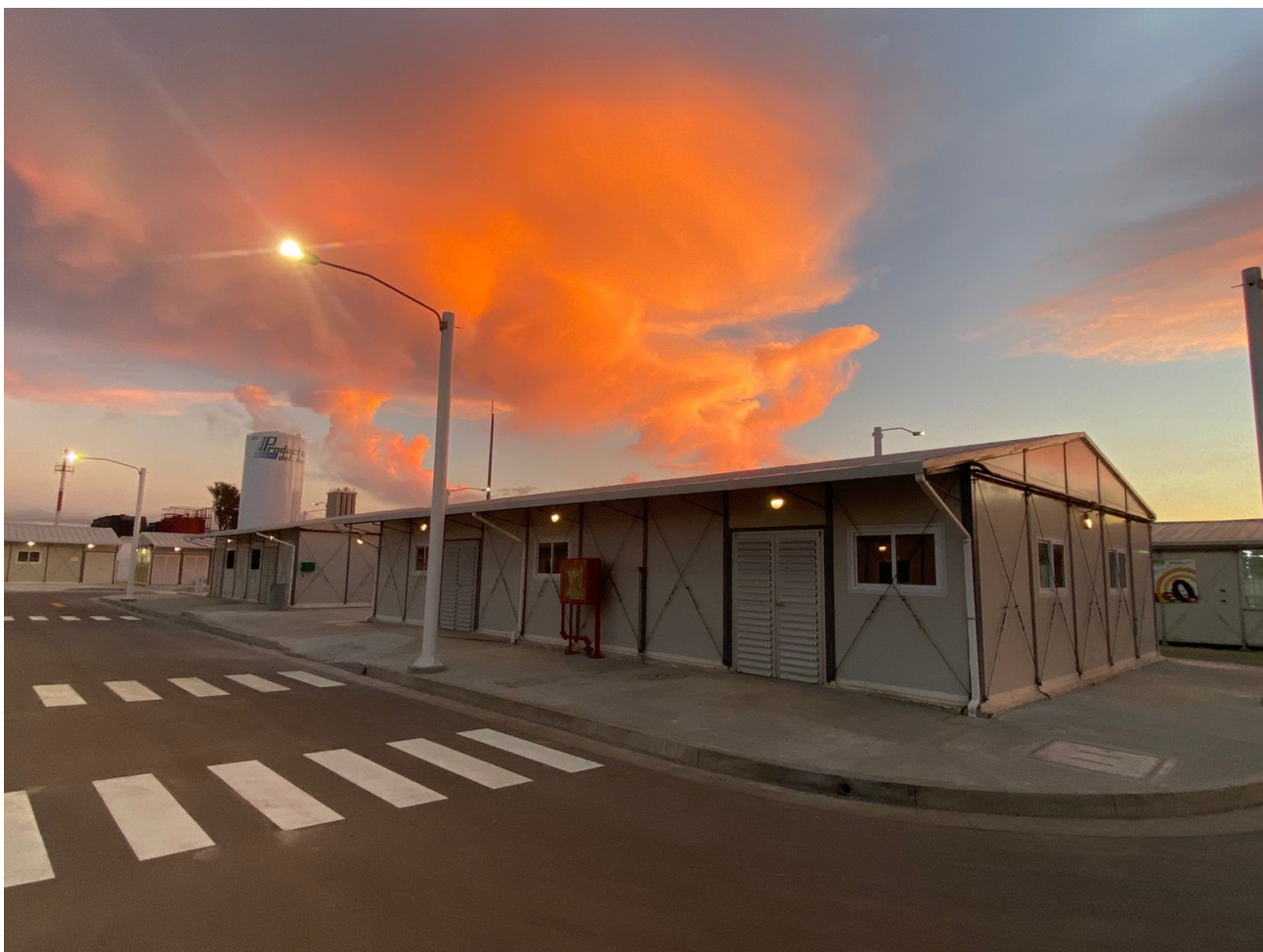
Hospital constructed by ATCO Espaciomovil - Escuintla, Guatemala
