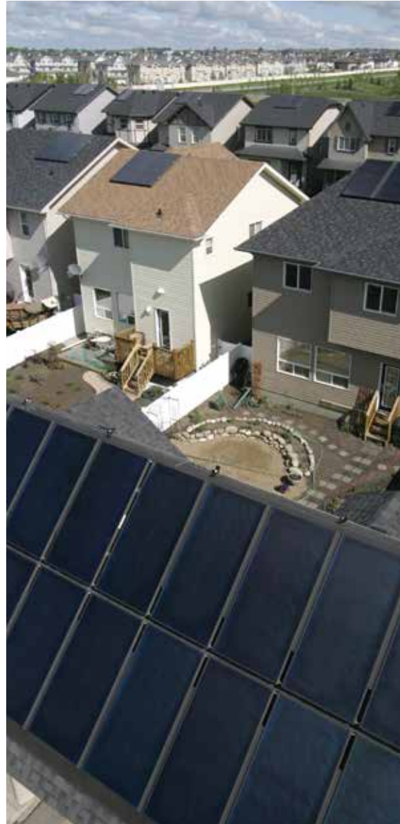
ATCO Gas helped develop and now operates the Drake Landing solar community in Okotoks, Alberta. The community set a new world record for energy efficiency and innovation by generating 97 per cent of its space heating needs through solar energy in 2011, earning a prestigious Energy Globe World Award.
