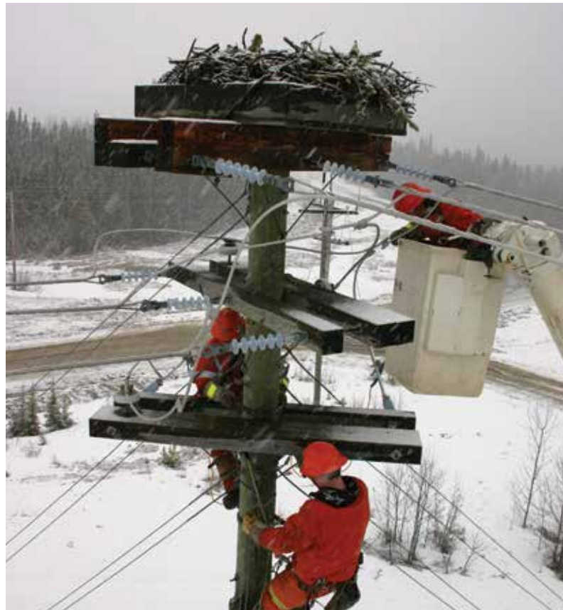
Ferruginous hawks (top photo) are a threatened species in North America. Their nests are accessible to predators, so ATCO Electric installs coyote-proof nesting platforms for interested landowners. Power poles are a prime site for huge osprey nests, but these nests cause problems for the birds and the equipment, so ATCO Electric builds nest platforms and carefully moves the nest to a safer home.
